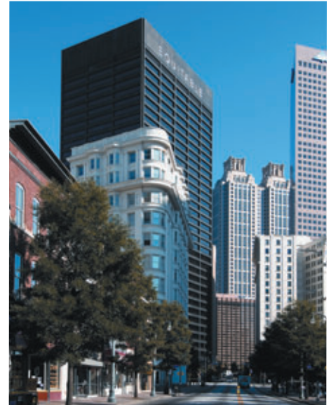
A landmark 33-story class A office building in downtown Atlanta, 100 Peachtree sustained damages from a tornado that tore through the city's central business district on March 14, 2008.
