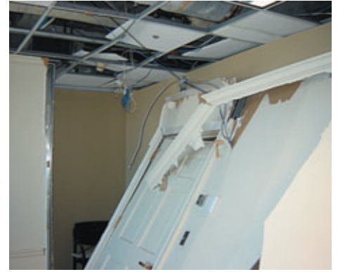
Damage to approximately half of 100 Peachtree's 44 tenants' spaces included fallen ceiling tiles, knocked-out interior walls, and broken windows. Floor plans and interior photos helped Equastone and EPIC Response expedite the damage assessment process and clear common areas quickly.
